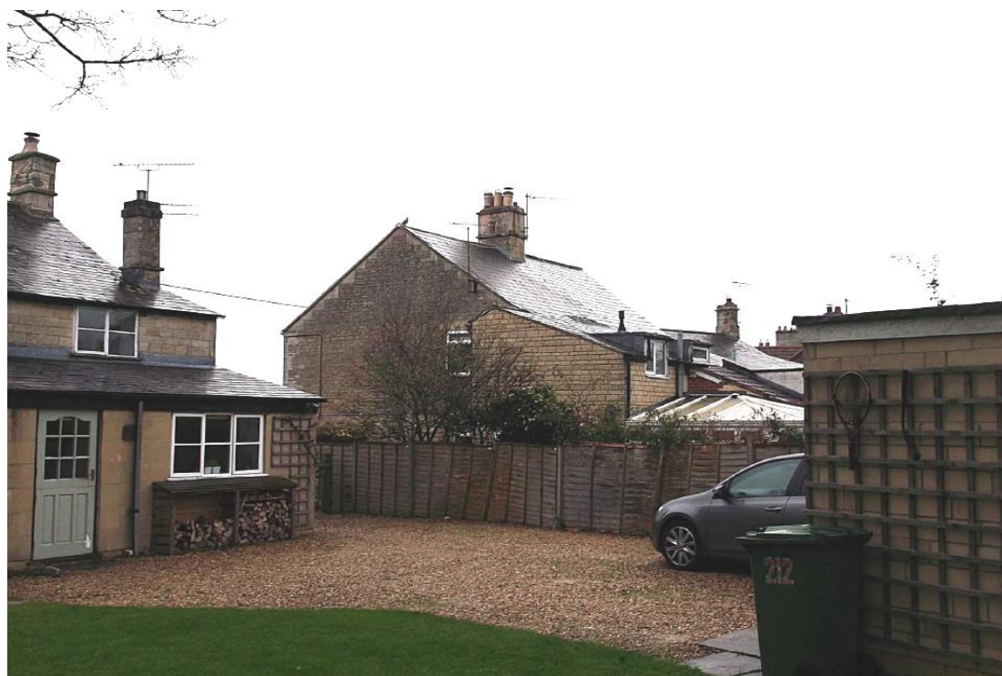
A view towards No. 211 (in the middle ground of the photo)
